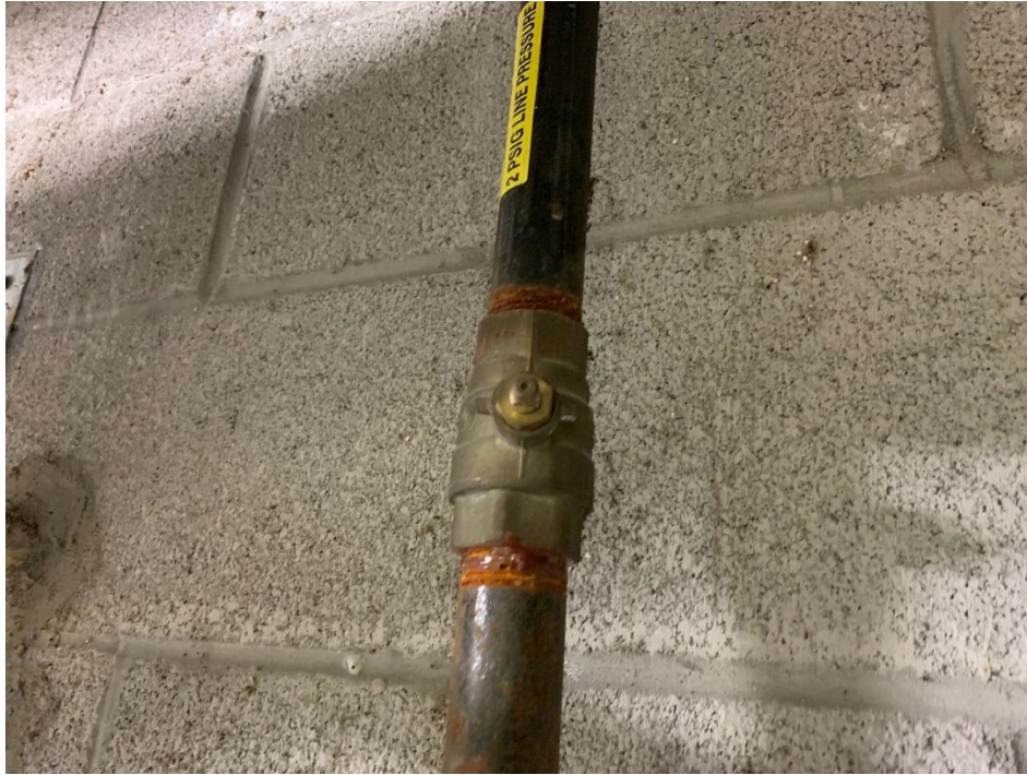
Gas valve shut off in Second Floor Mechanical Rooms but still connected to individual rooms.
