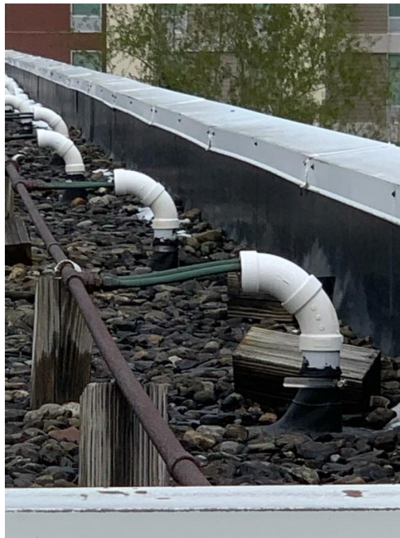
Unsealed Header Pipes
