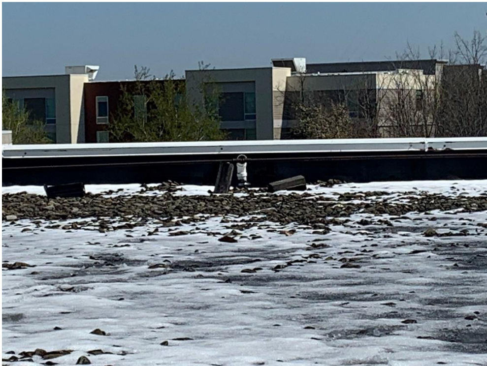
Gas header pipe on roof with support falling off
